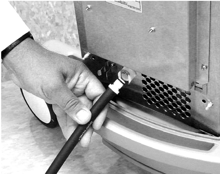
Figure 7.3. Push Hose Into Drain Coupler
